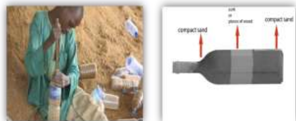
Fig. 5 Method of filling the plastic bottles for using in the building
