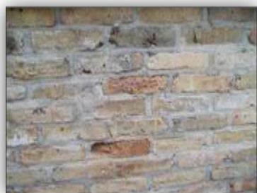
Fig. 6 Brittleness characteristic of the brick
