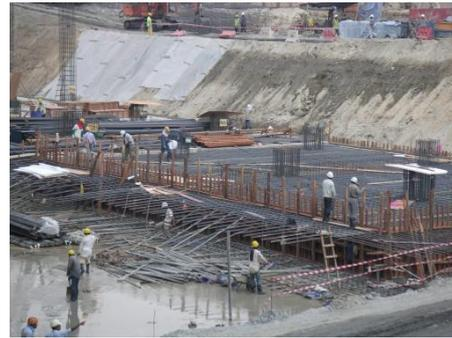
Fig. 7b: Construction of raft foundation
