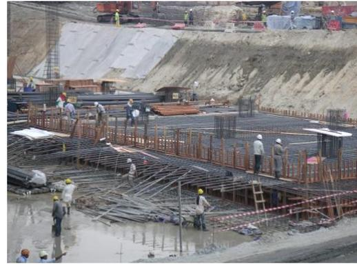
Fig. 12: Strip/pad footings under construction Fig. 13: A raft Foundation under construction
