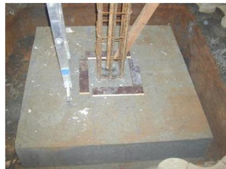
**Fig. 11:** A pad footing under construction
