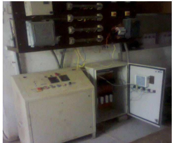
Fig.3- Designed and Commissioned APFC at Arihant Marble Industry
