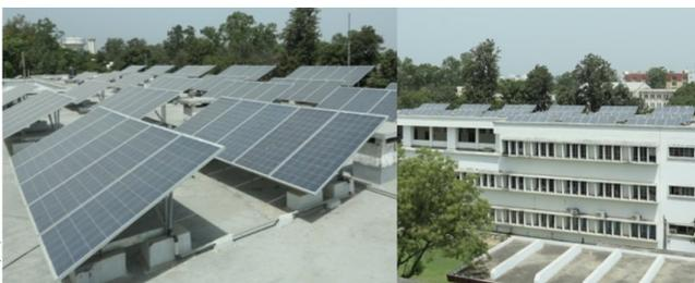
Fig. 3. SPV modules with a tilt of 25 degrees mounted on roof top of Reference Building
