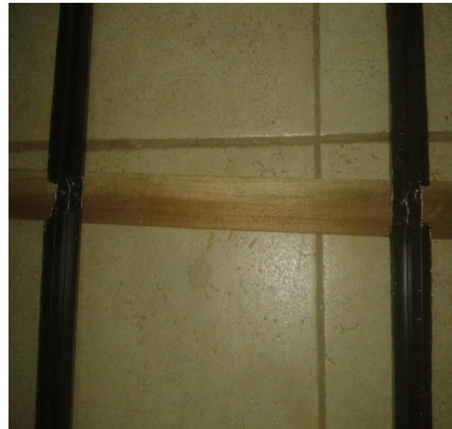
Figure 5. Showing the Crack in the Railway Track
