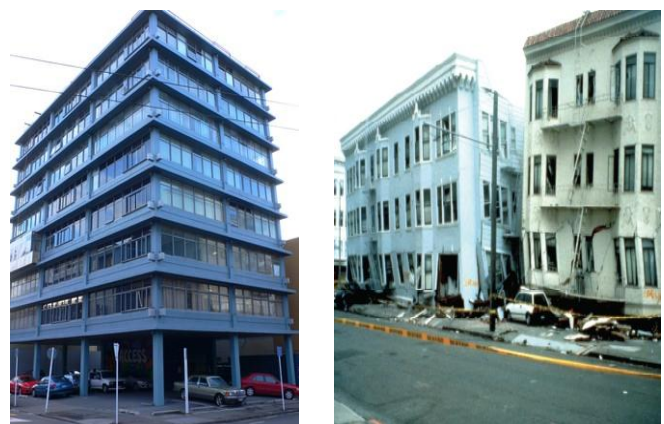
Fig 1. Soft Storey Building (Left side) and Collapsing of open ground floor (Right side)
