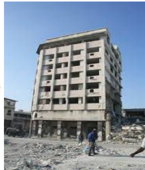
Fig 1.2 Actual view of multistorey building with soft storey
